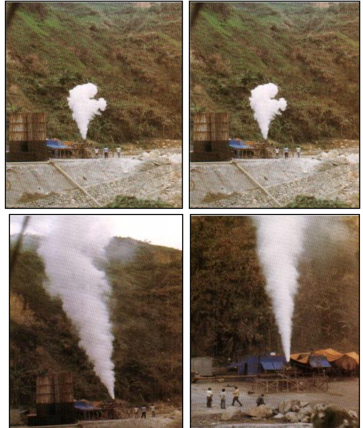
Drilling of Exploratory Well AC-1D
