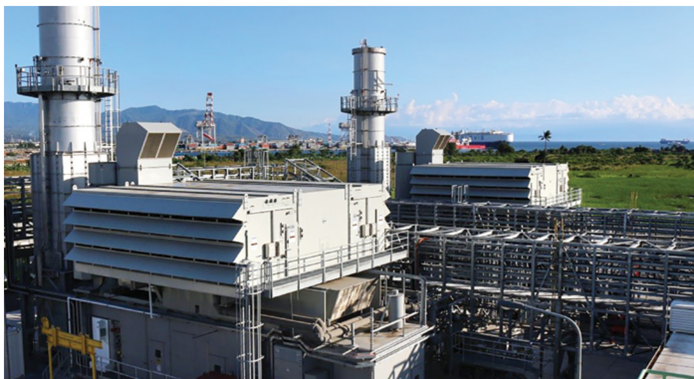
Figure 13. Prime Meridian Powergen Corporation's (PMPC) 97 MW Avion Open-Cycle Natural Gas-Fired Power Plant which started commercial operations on September 26, 2016 in the First Gen Clean Energy Complex in Batangas City.
