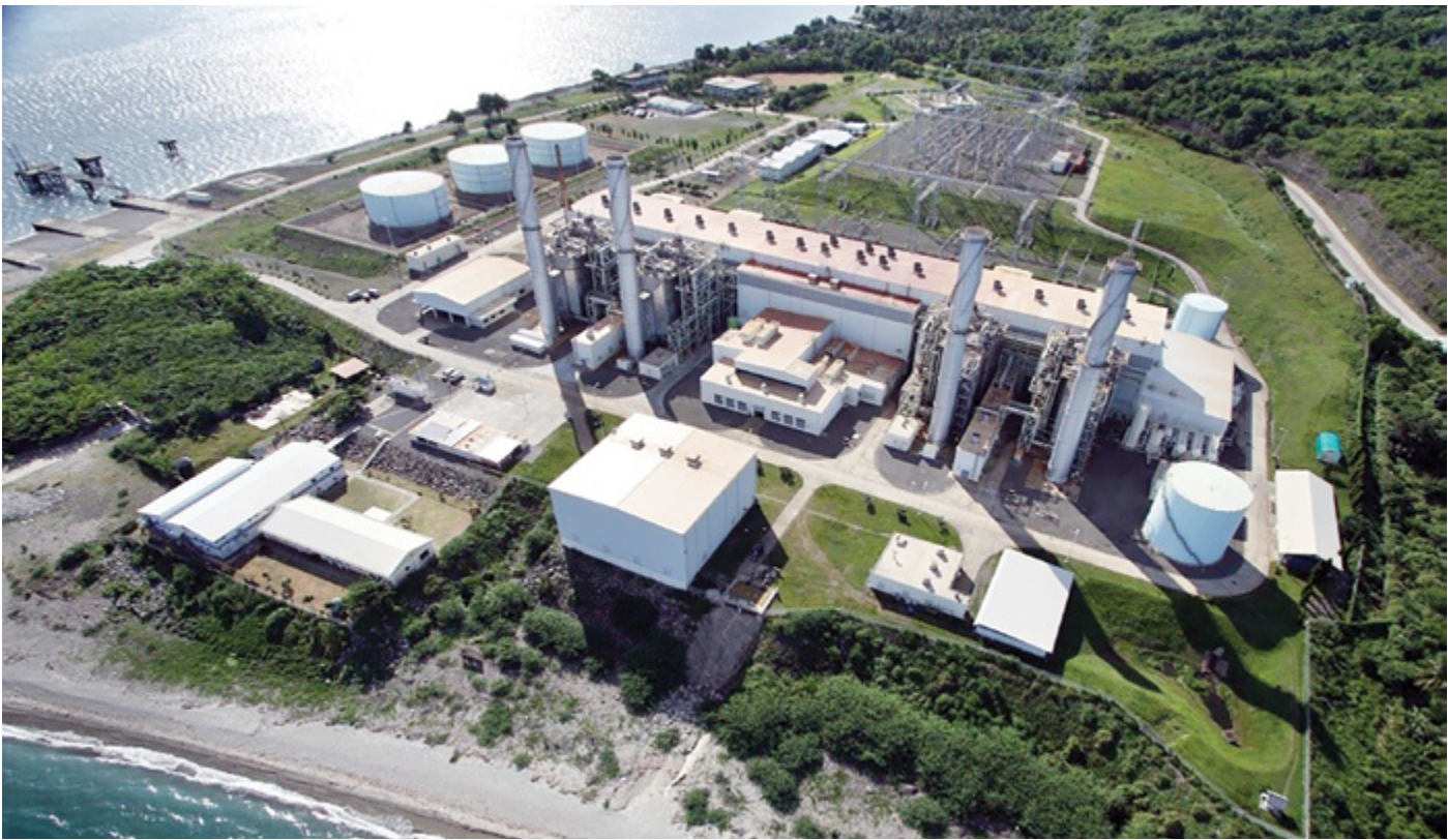
Figure 14. The 1,200 MW Ilijan Combined-Cycle Power Plant, the largest natural gas facility in the country, is being operated by KEPCO Ilijan Corporation (KEILCO) in Ilijan, Batangas.
