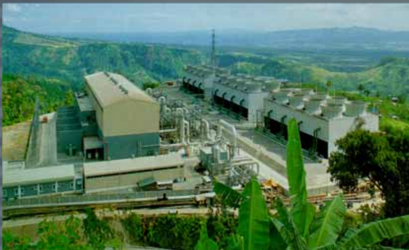
Malitbog Facility in Leyte: Largest Geothermal Field in the World
