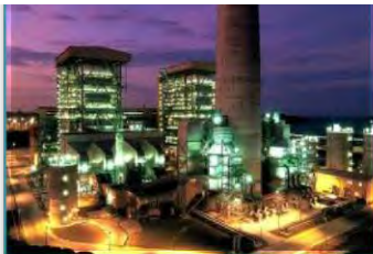
1294 MW Sual Coal-fired Power Plant
