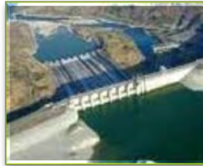
360 MW Magat Hydroelectric Power Plant
