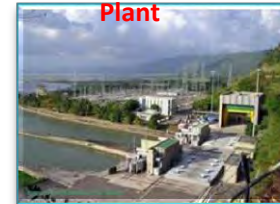
755MW CBK Hydroelectric Power Plant
