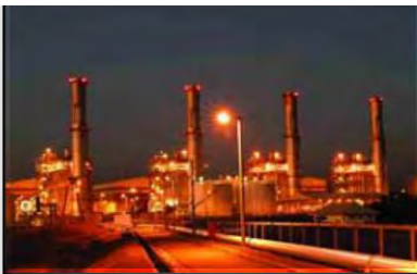
Sta Rita Natural Gas-fired Plant
