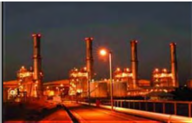
1060 MW Sta Rita Natural Gas-fired Plant
