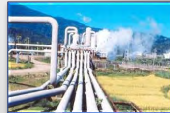
610 MW Leyte Geothermal Power Plant
