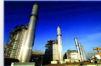
500 MW San Lorenzo Natural Gas-fired Plant
